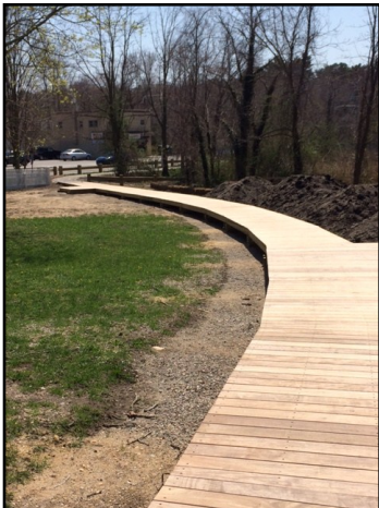
New boardwalk from Swezey-Avey House to spillway under construction
