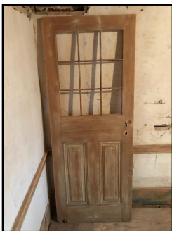
Original doors are being sanded, repaired, and painted prior to installation.
