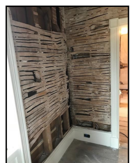
Original lath will be retained wherever possible.
