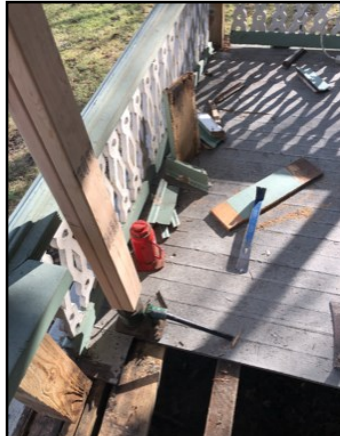
Repairs to the Hawkins House front porch. Rot and insect damaged areas are being completely replaced. Jeremiah McGiff, Restoration Carpenter, is heading up this project.
