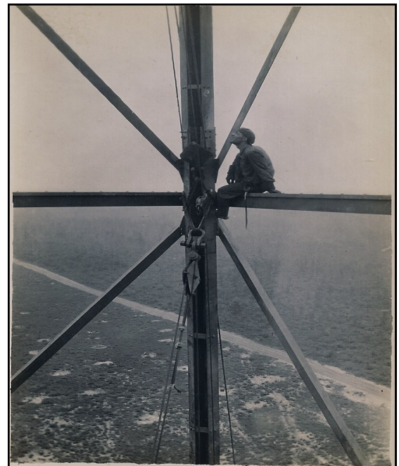
Attaching blocks to tower
